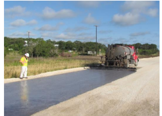
Terra Prime TM application in Florence, Texas
