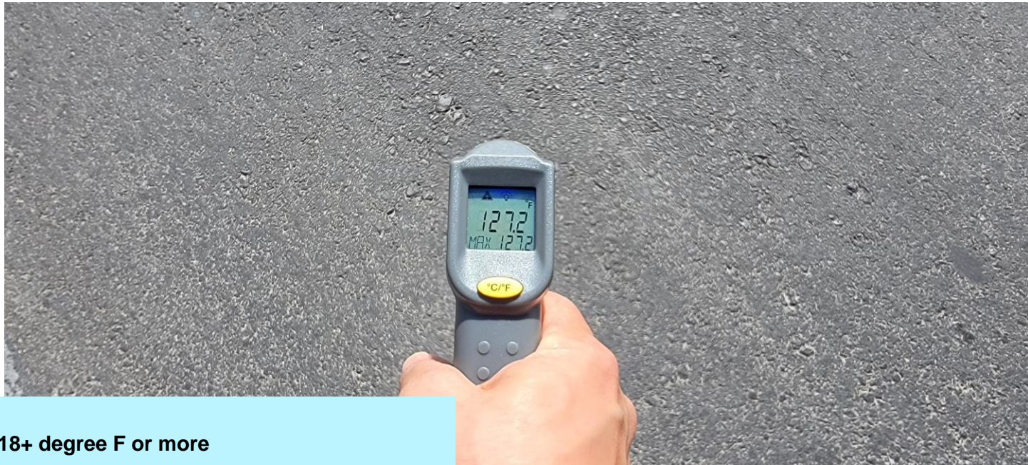
Asphalt Surface @ 127.2 degrees F
